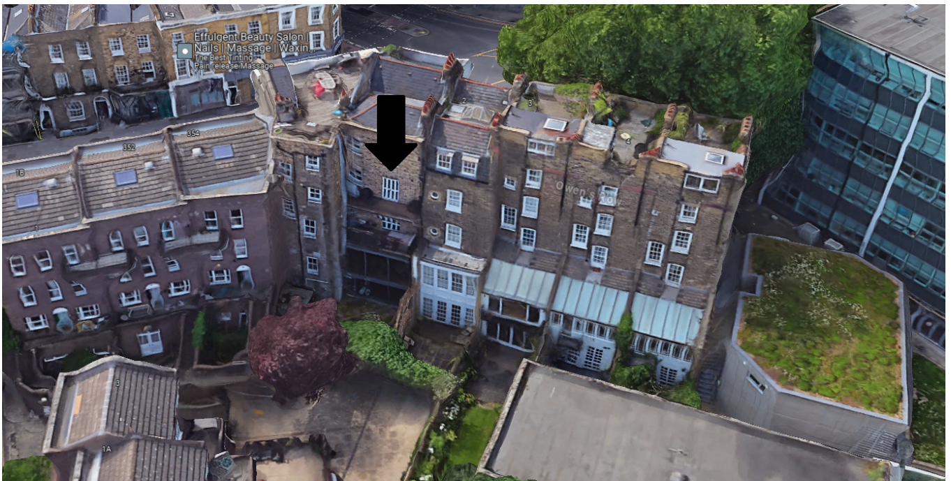
Image 3: Aerial View of the rear of the site within wider site context
